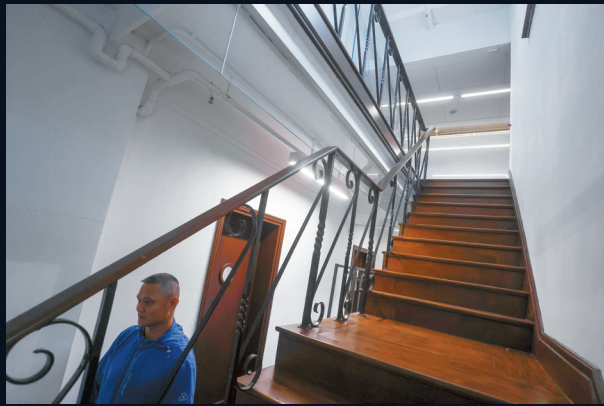
The original timber staircase in Block A.
