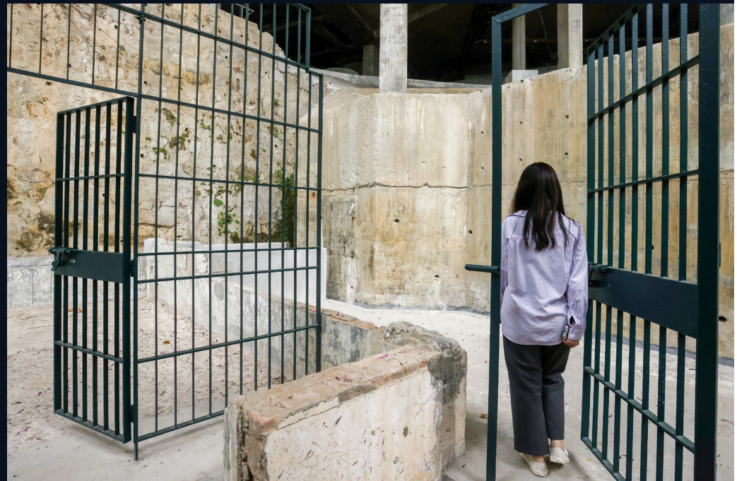
The jail cells in Block C at the former Victoria Road Detention Centre.
